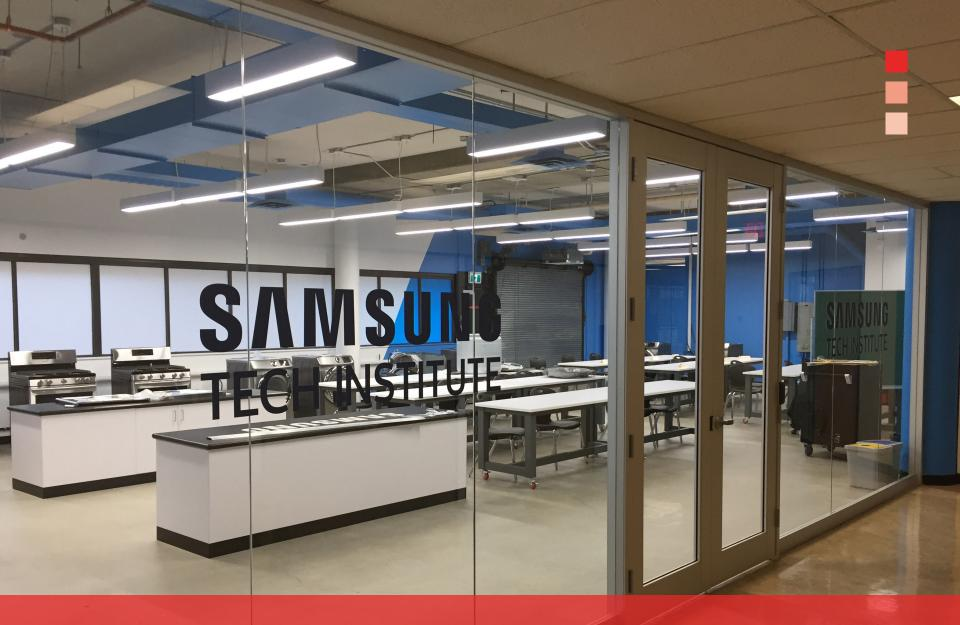
Classic stick-built glazing allows you to partition off workrooms and offices while maintaining an open floorplan and uninterrupted flow of light. Sturdy double aluminum doors can be combined with butt-jointed glass for a continuous effect.
